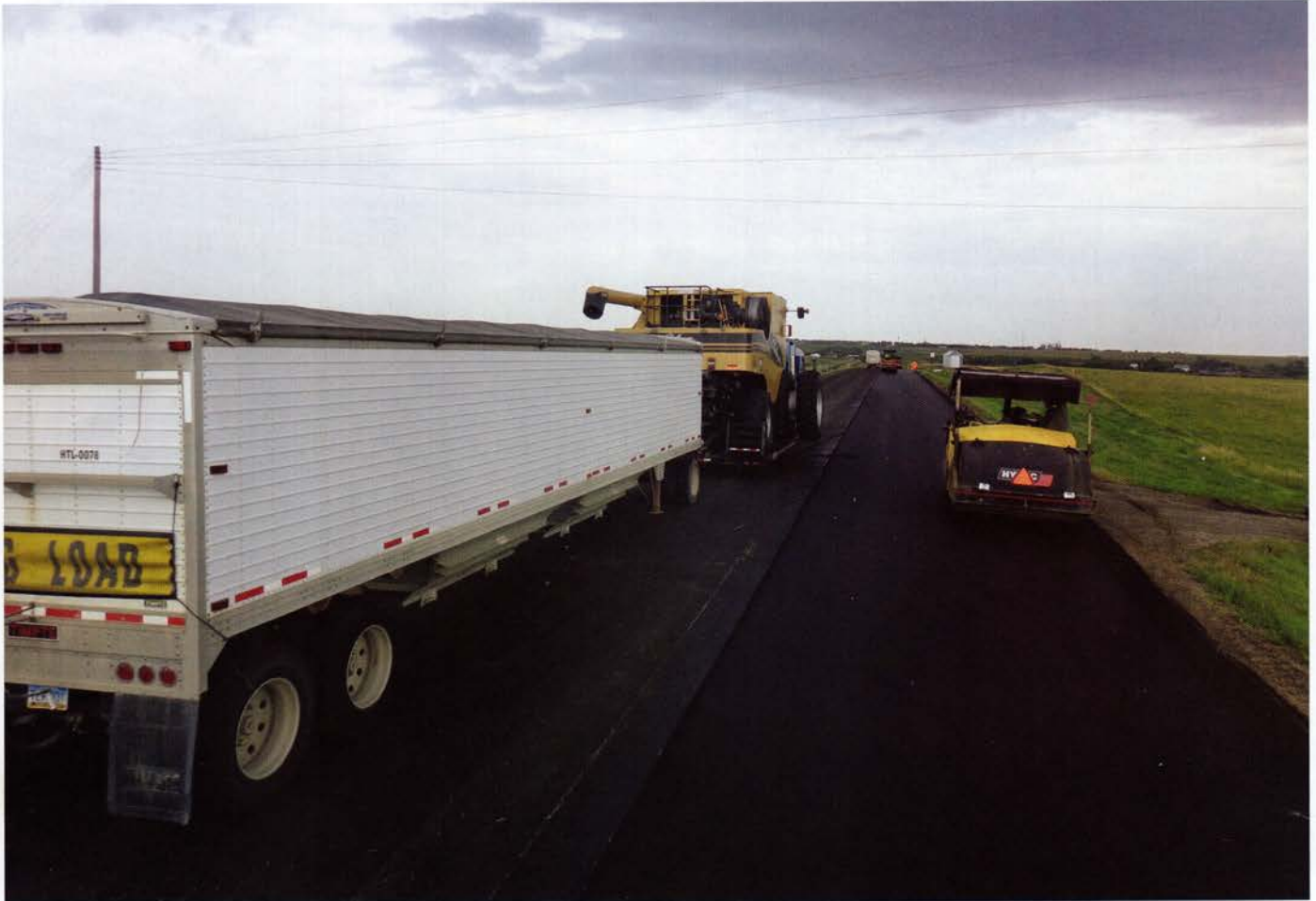
The traffic out on the plains is a little different than that you experience in urban paving zones. Farming equipment and trailers filled with corn went by on occasion. You can also see the compaction team in this picture. Looking from the back of the paver, you can see the Hypac in breakdown position. The Dynapac machine is the intermediate roller.
