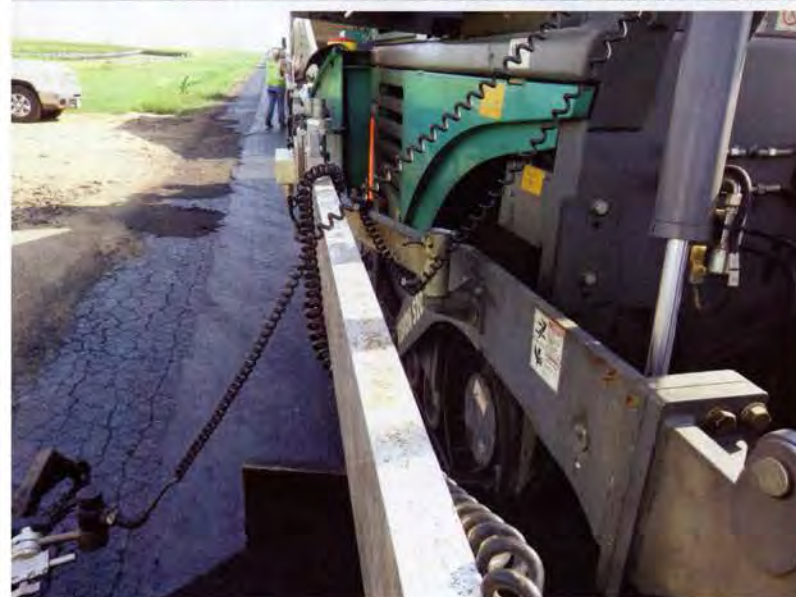
TOP: The Topcon ski is out about 2 1/2 feet matching the joint on the new mat. The material is about 1/2-inch above the joint for perfect compaction to take place. The guide bar is out for the paver, which is paving 14 feet wide. The endgate is tight to the edge. It's a different apparatus from the MOBA device, which is on the other side of the paver. BOTTOM: The crew ran MOBA technology on the other side of the machine. This ski is 30 feet long and on the side of the road that is rough. We didn't want to match the rough edge, of course, so we kept the ski close to the paver.
