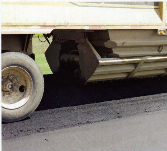
LEFT: This is the truck depositing the mix. They don't open the belly dump any further than this. They'll end up with too much mix on the ground and it'll overflow the paver if they open it too far. It takes years of practice and experience to get this just right. RIGHT: 25 tons of mix runs out about 190 feet. At each connection, there'll be tire marks where the finished truck pulls away. Look at the mud flaps providing a nice V shape. The trucks have two chambers in them.
