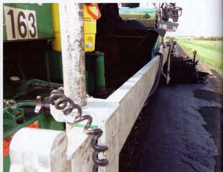
TOP: The Topcon ski is out about 2 1/2 feet matching the joint on the new mat. The material is about 1/2-inch above the joint for perfect compaction to take place. The guide bar is out for the paver, which is paving 14 feet wide. The endgate is tight to the edge. It's a different apparatus from the MOBA device, which is on the other side of the paver. BOTTOM: The crew ran MOBA technology on the other side of the machine. This ski is 30 feet long and on the side of the road that is rough. We didn't want to match the rough edge, of course, so we kept the ski close to the paver.
