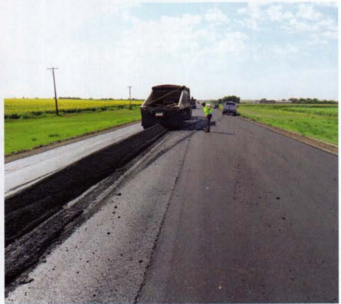
LEFT: This is the truck depositing the mix. They don't open the belly dump any further than this. They'll end up with too much mix on the ground and it'll overflow the paver if they open it too far. It takes years of practice and experience to get this just right. RIGHT: 25 tons of mix runs out about 190 feet. At each connection, there'll be tire marks where the finished truck pulls away. Look at the mud flaps providing a nice V shape. The trucks have two chambers in them.
